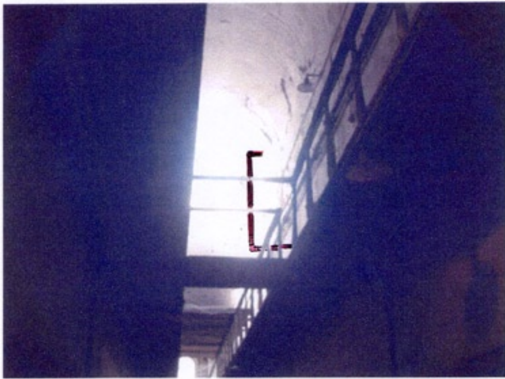
View from CB 4 1st floor facing North
