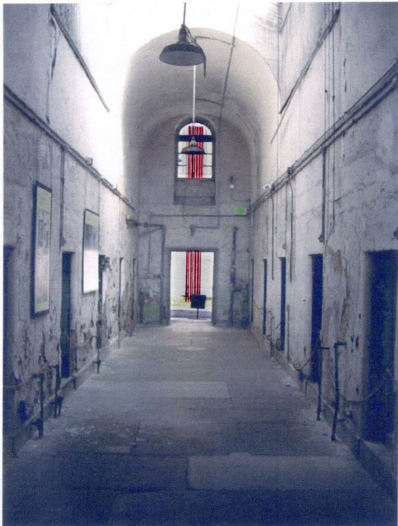
view from CBZ corridor.
