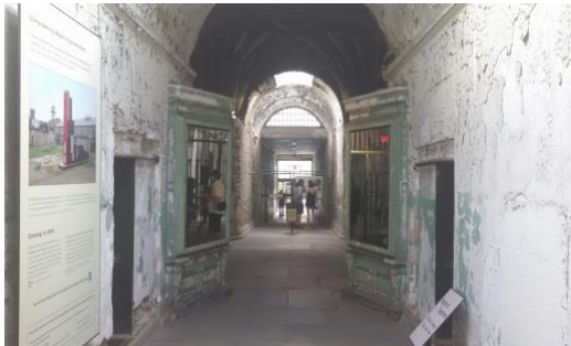
Surveillance Mirrors and Cell Block Expansion
