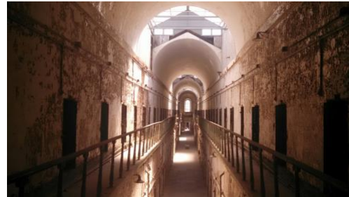
Two-Story Cell Block with Barrel Vaulted Ceiling
